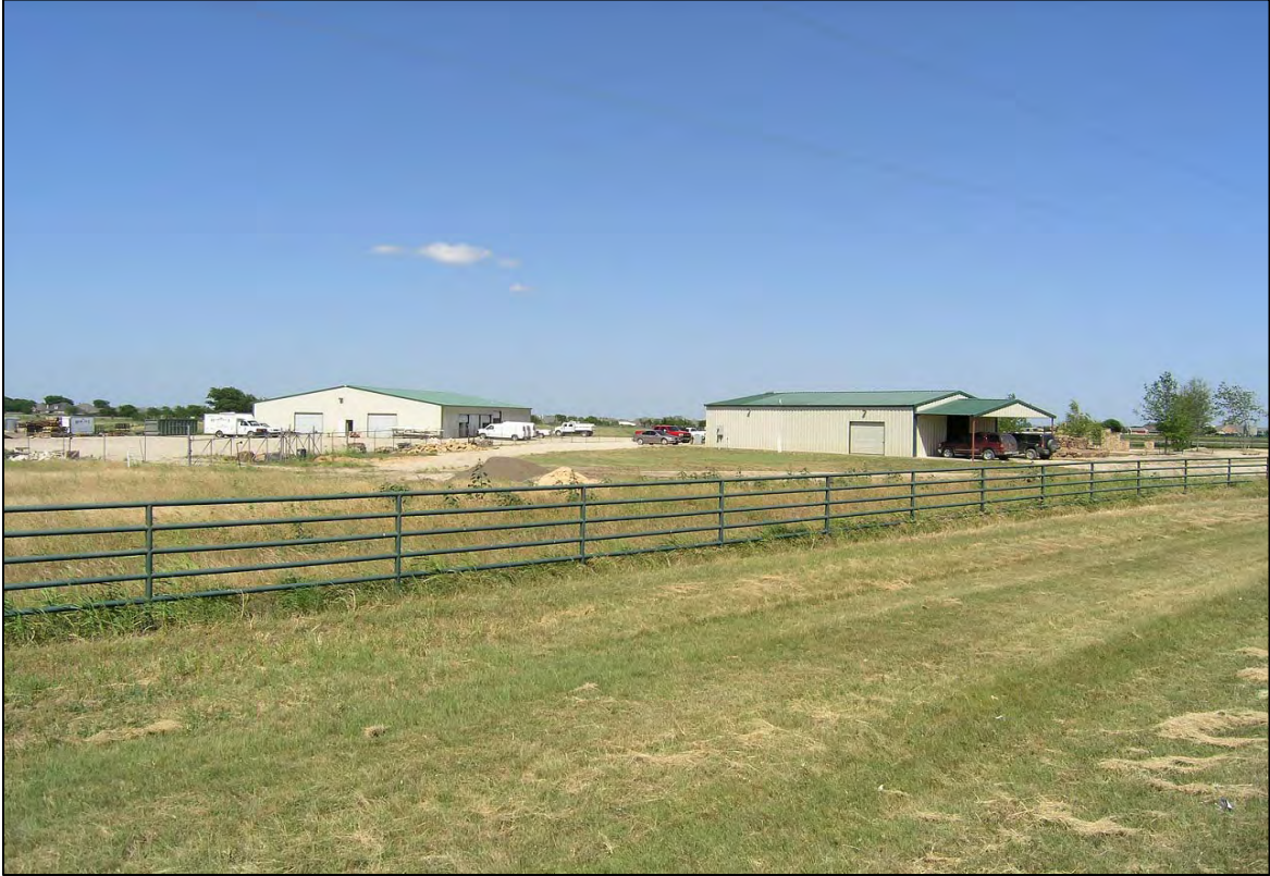
Buildings - Frontage Road View
