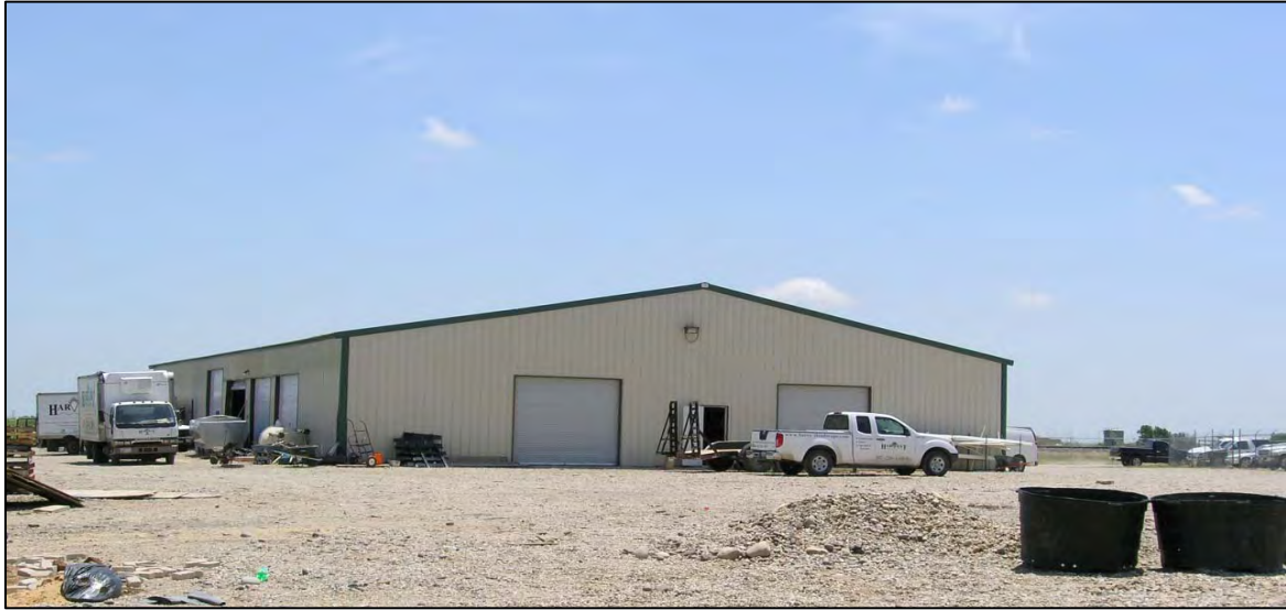
Warehouse Bldg - Side View
