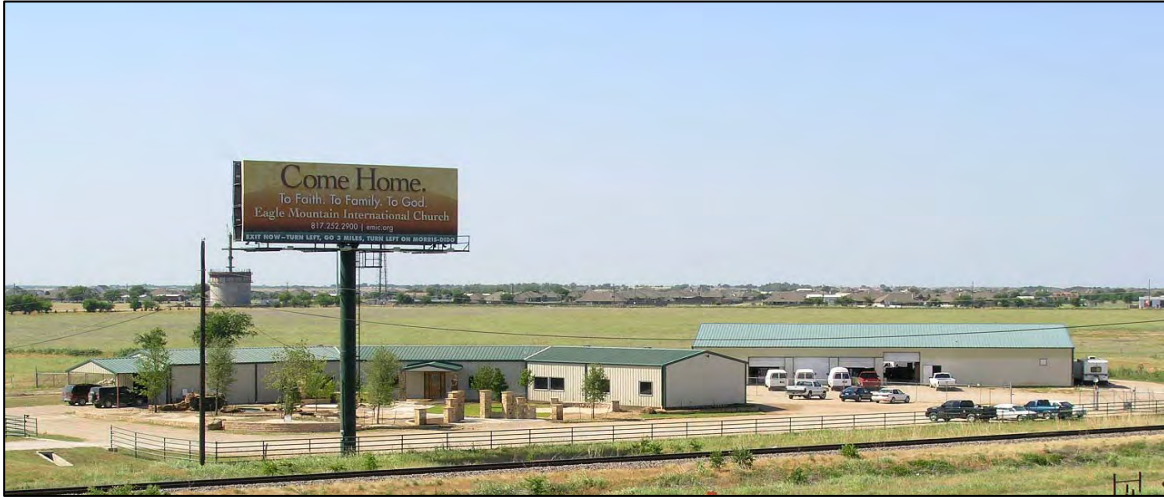
Buildings - Highway View 1
