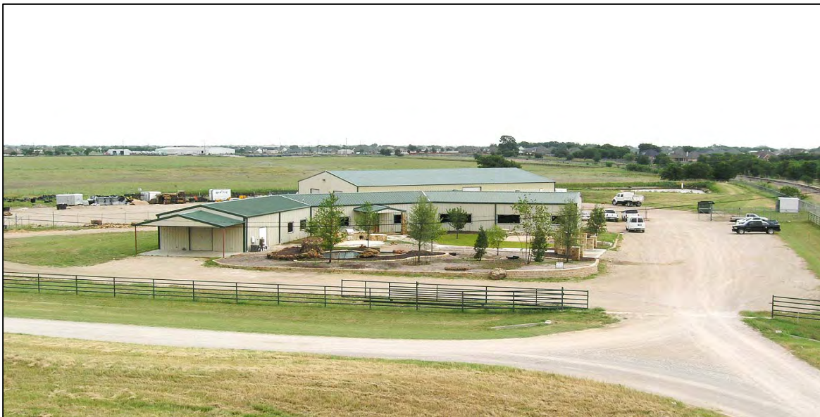
Buildings - Highway View 2
